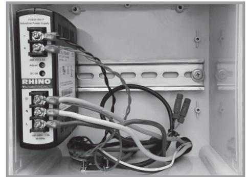
Location of float switch connection leads in controller box.
