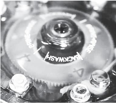
C. Check the meter disc under the amber cap on the softener control valve. If the proper meter disc is not already installed in the system, you'll replace it with the appropriate numbered disc located in the installation kit using the following steps:
